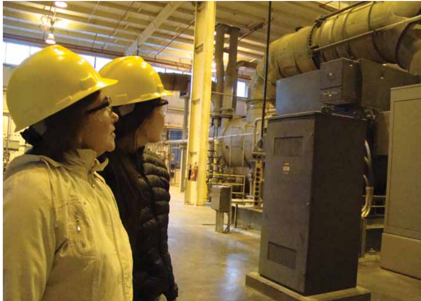
Tatiana Tivikova (left) and Galina Angarova tour the Calpine geothermal plant in Middleton, California
